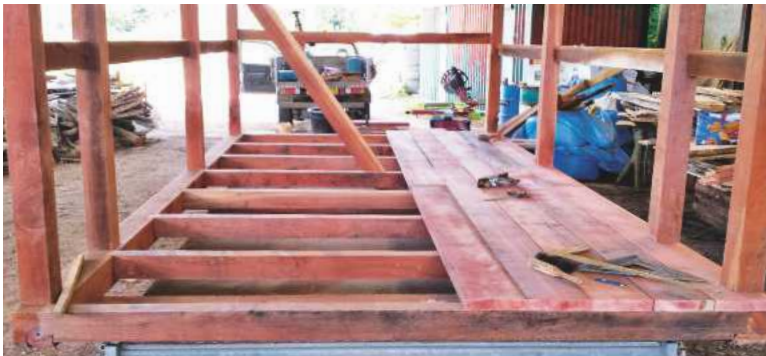
The basic frame is constructed on its trailer
